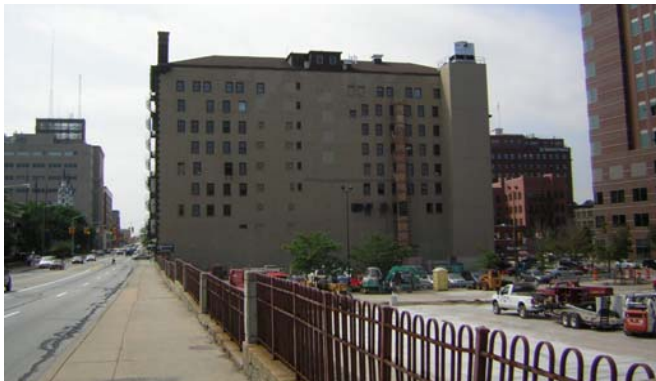
View of existing parking lot looking south to the Commerce Building
