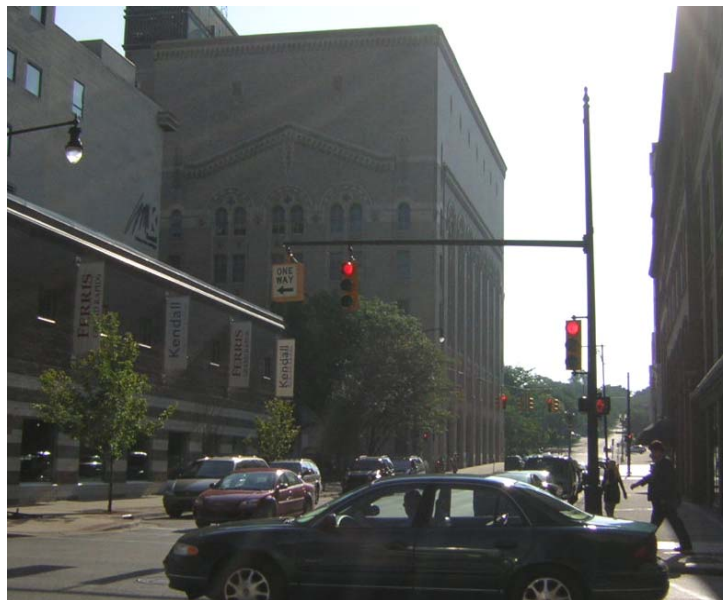
Existing view looking east up the hill on Fountain Street towards the ATC
