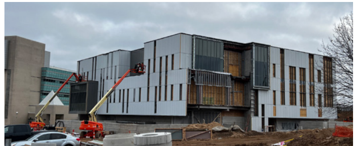
CONSTRUCTION IN PROGRESS, TAKEN 12.13.22
