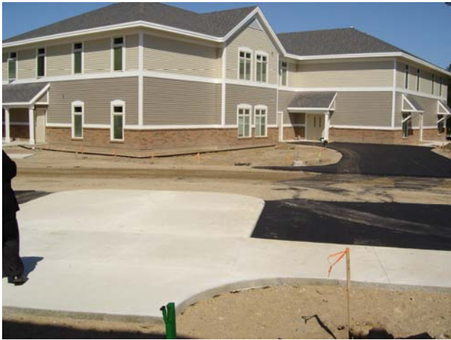
Lighthouse Academy in its final stages of construction in late August
